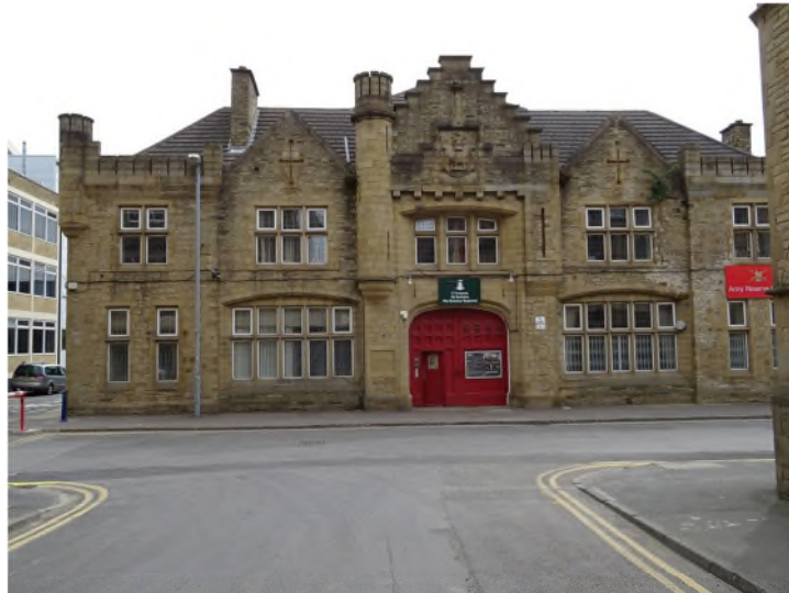
Huddersfield Drill Hall, St Pauls Street
